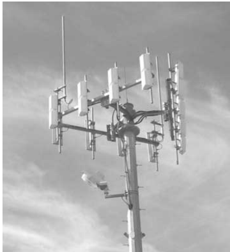
Figure 16.5 Sectorized base-station antenna.
